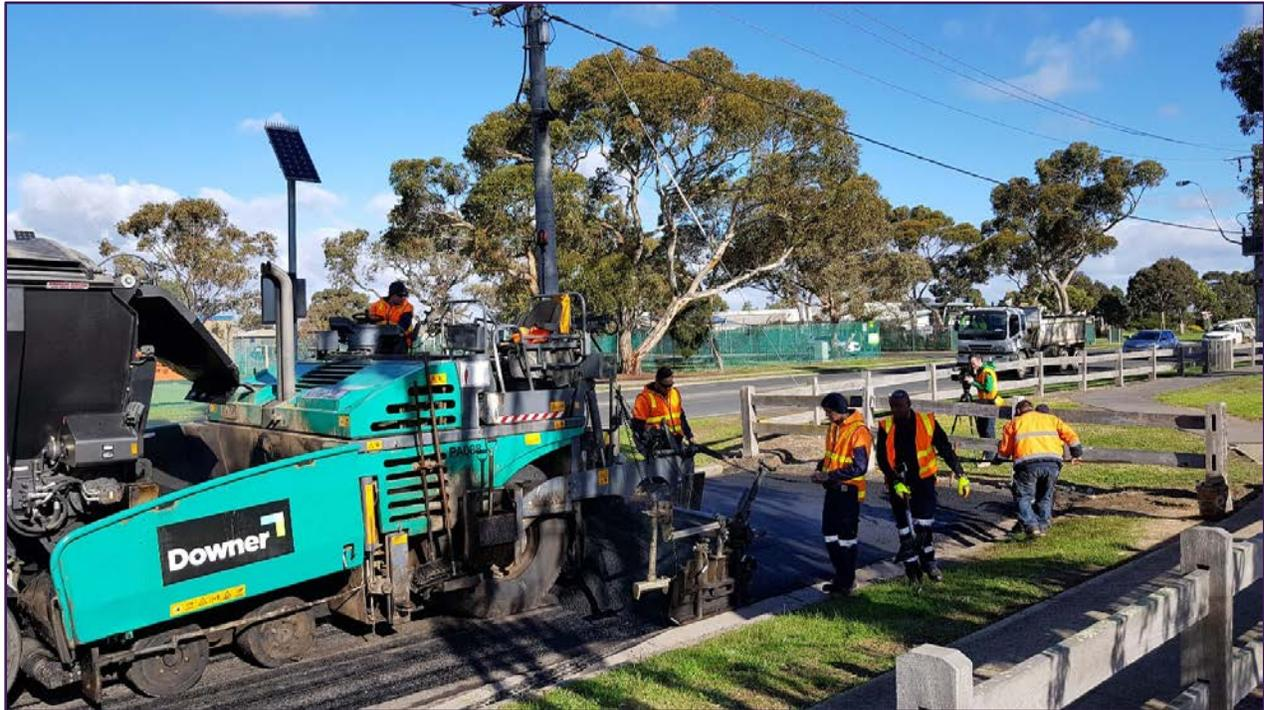
*Photo of the road reconstruction process supplied thanks to Downer*
